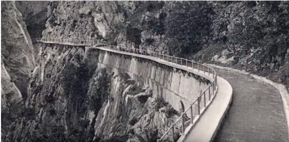
In order to maintain the older dam and the canals, and to control the flow of water with special gates, a trail was constructed along it.
