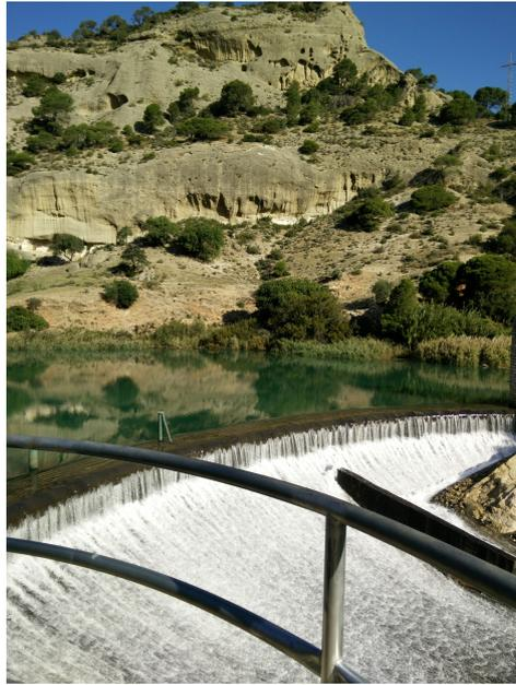
The lower dam, built in 1903-1905, diverted the water into tunnels and canals, with a total length of 3 km.
